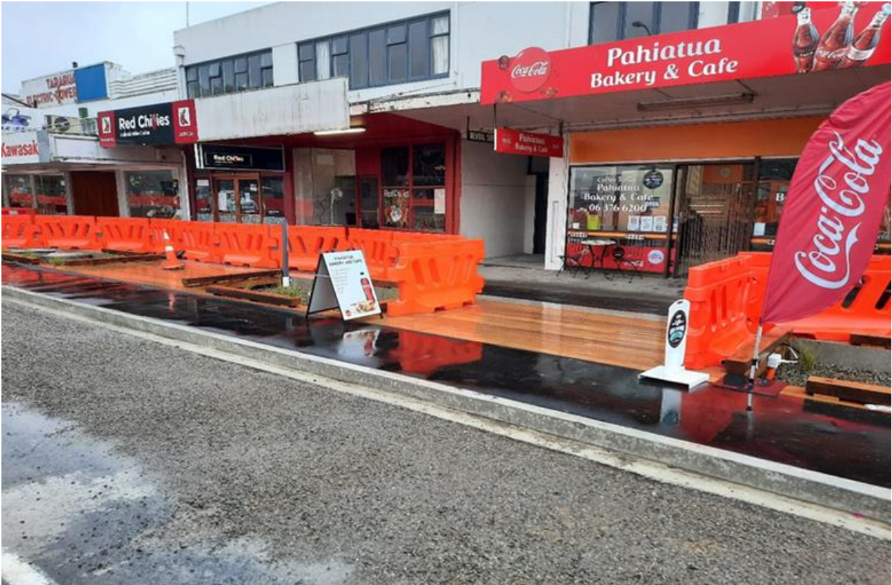
Bio-filter garden and footpaths nearing completion
